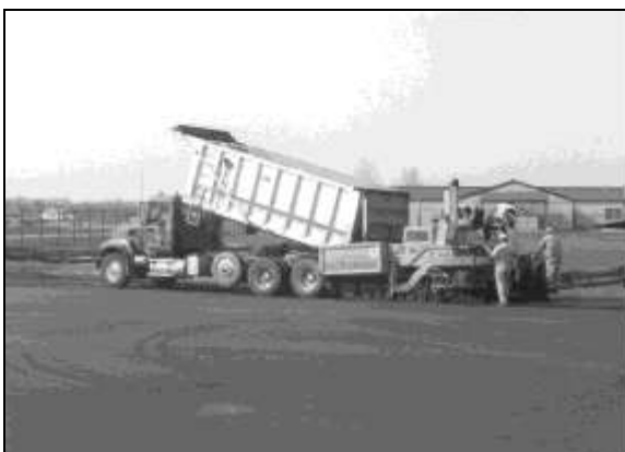
Construction of the ramp addition
